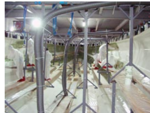
Application of Scott Bader Barrier Coat
